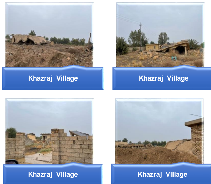
Picture 2 The destroyed houses from Khazraj, Sayed Gharib Village
